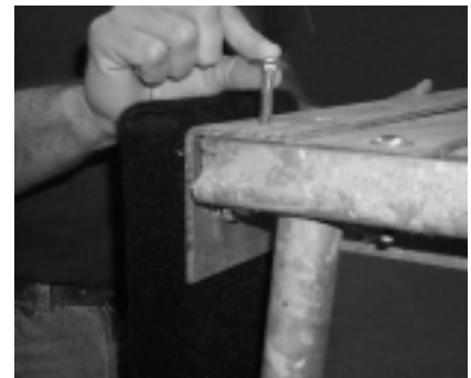
18. Secure the dock mounting angle (Ref.#20) onto the dock with three (3) 5/16" X 2-1/4" carriage bolts (Ref.#29) and three (3) 5/16" hex nuts (Ref.#40).
