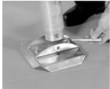
3. Mount the adjustable leg to the base pad channel using a 1/2" X 4-1/2" hex bolt and secure with a 1/2" flange lock nut.
