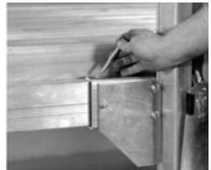
18. Mount the entire hoist by sliding the winch post mounting channel over the dock mount tube and drop two 3/8" X 3-1/4" hex bolts down through holes on winchpost mounting channel to secure the hoist to the dock.
